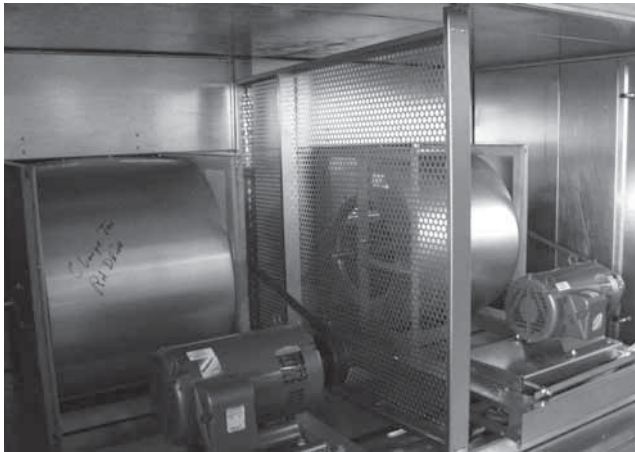
Figure 1 – SWSI dual fan segment (Inlet side shown)
